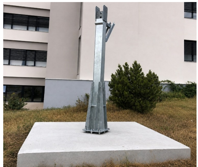
Fig. 15 Concrete foundation and installing vertical steel pole
